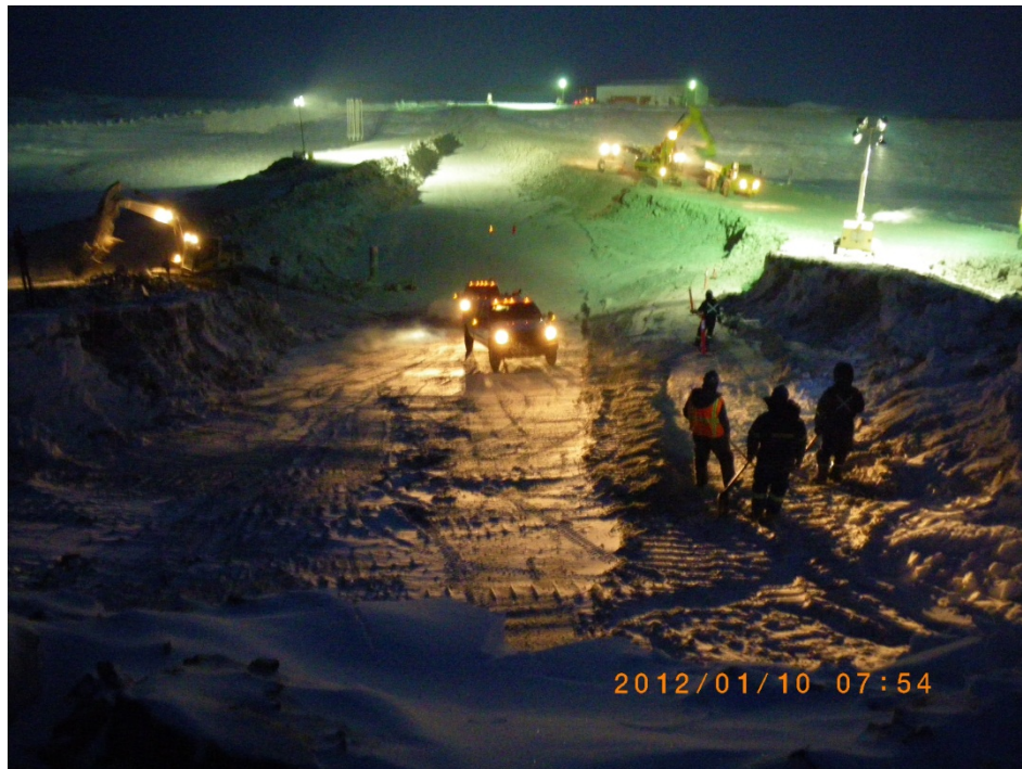
Photo 1: In the foreground, an attempt to expose the damaged liner, by hand, was unsuccessful as the material over the liner was frozen.
