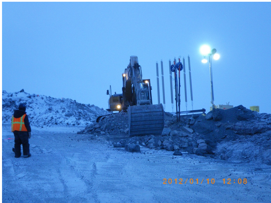
Photo 2: Careful excavation around the ground temperature cables at the west end of the key trench. Final excavation was completed by hand and the steel pipes housing the cables were carefully laid onto the base of the key trench.
