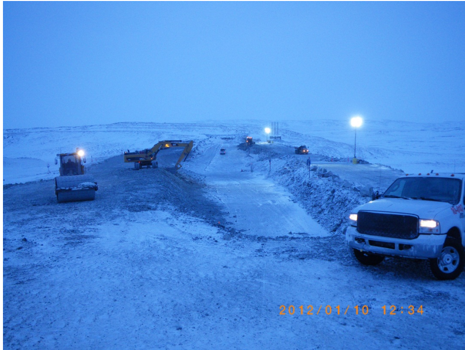
Photo 3: Removal and relocation of the protective material continues. The 10 tonne compactor works the ROQ surface within the upstream ROQ shell of the dam
